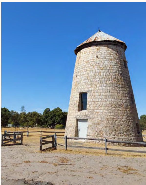
ABOVE: Inlet Park and Chapman's Mill, Reinscourt P421
